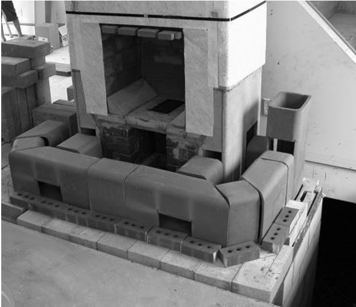
Figure 3. Dry Heated Bench layout and chimney connection
