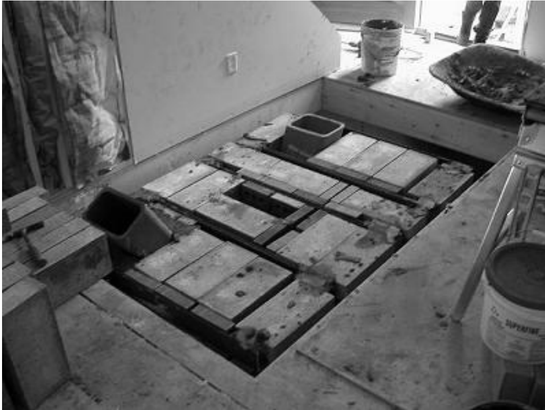
Figure 2. Chimneys coming up through foundation.
