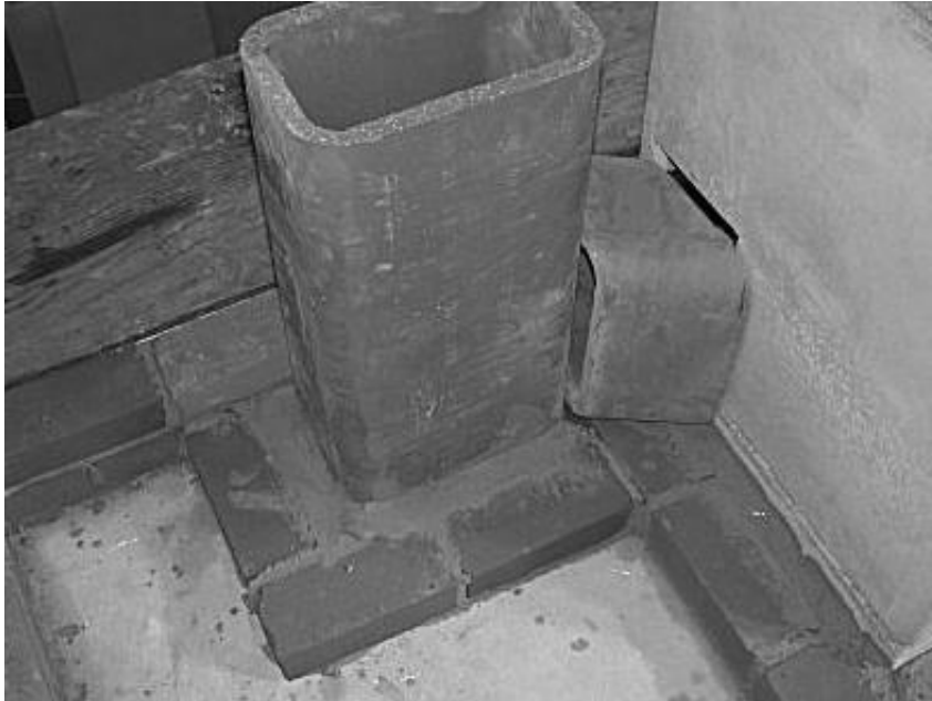
Figure 4. Chimney Connection.
