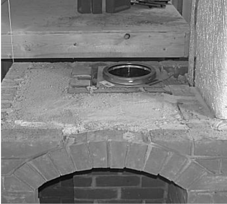
Figure 6. Metal chimney connection
